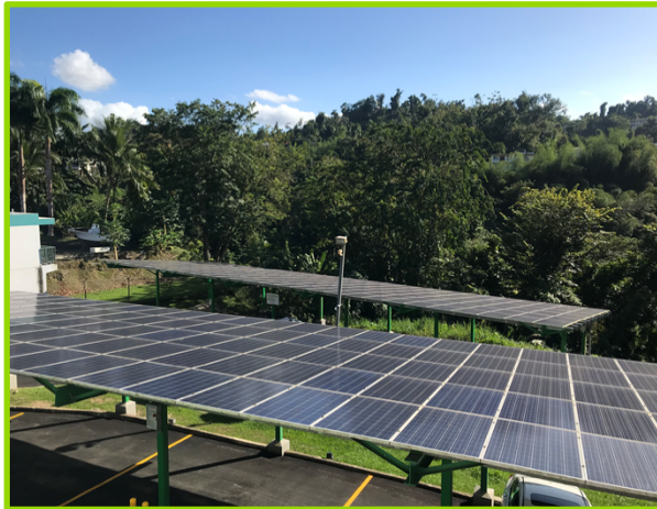
Solar carports at Cooperativa Jesús Obrero’s Guaynabo location provide electricity for the building.
