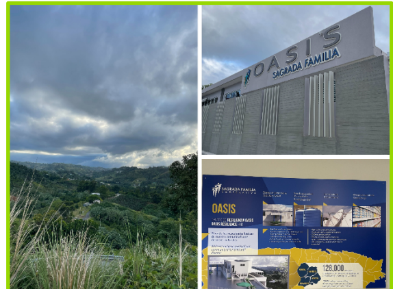
Cooperativa Sagrada Familia's branch in Naranjito, Puerto Rico (top left) constructed an "Oasis" Resiliency Center (top right) that provides a central hub for hurricane resilience and response efforts – including fuel reserves, a kitchen, and satellite internet connection (bottom right).
